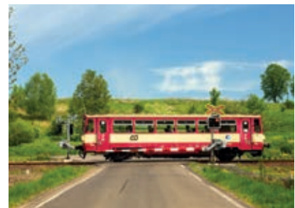
New installation of PZZ-RE level crossing from AŽD production on line Rakovník – Bečov nad Teplou.
